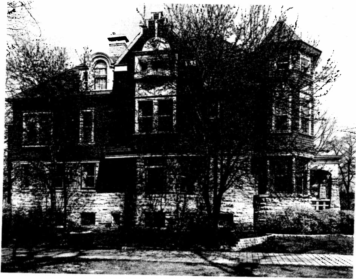
The Beeson House employs a variety of materials (stone, wood shingles, pressed metal), classically inspired details (broken pediments, Palladian windows), and unusual features (stepped gable, tiny balconies, overscaled keystones)—all befitting the eclectic Queen Anne style.
